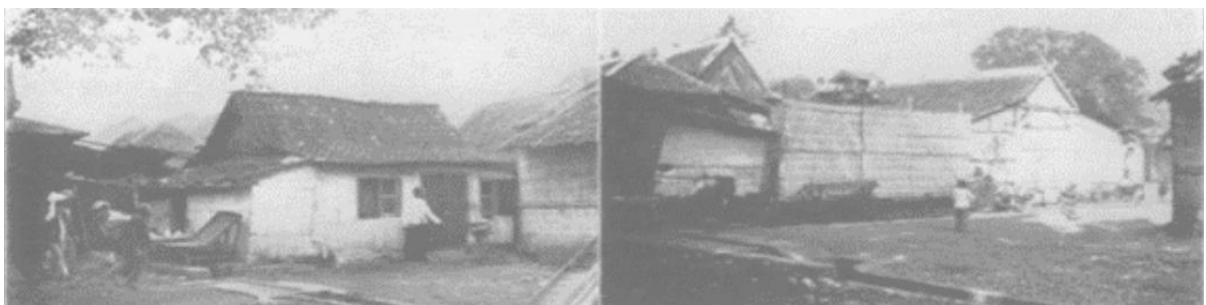
Picture 3. The process of demolishing indigenous houses in the implementation of the kampongverbetering program in 1930 (Source: (Flieringa, 1930))
