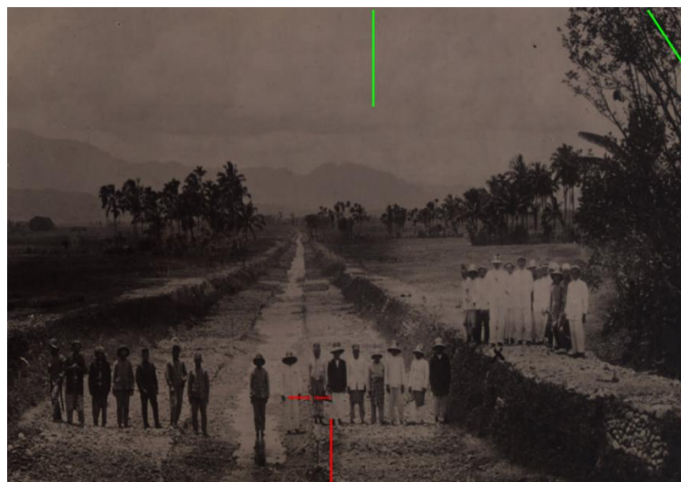
Figure 4. irrigation construction (KITLV, 1918)
